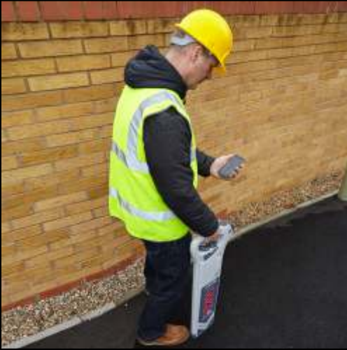
Acquire Utility Scan Data With GPS Overlays Of Survey Conducted
